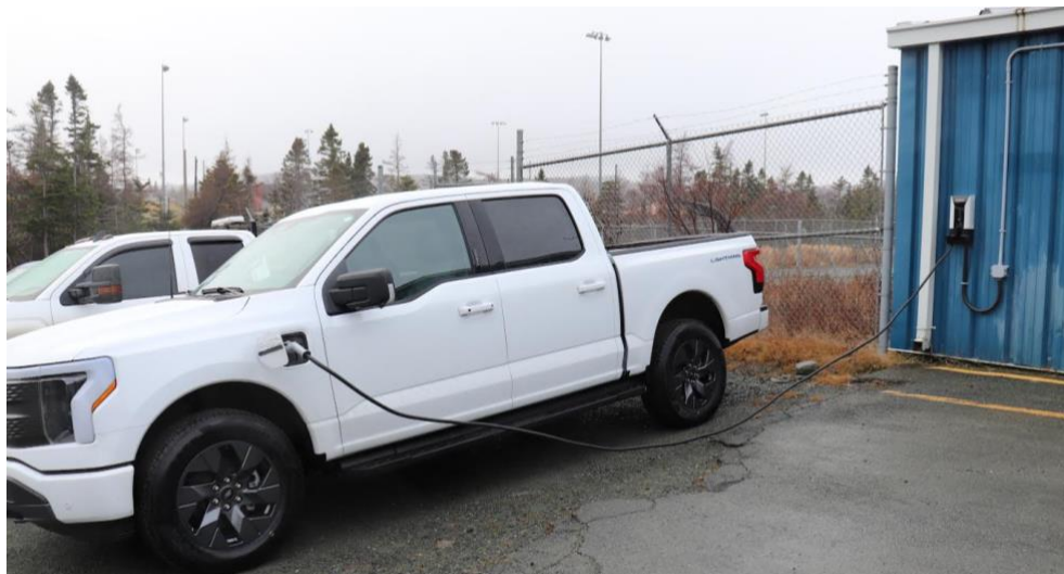
Figure 2.4 EV Charger Cables
