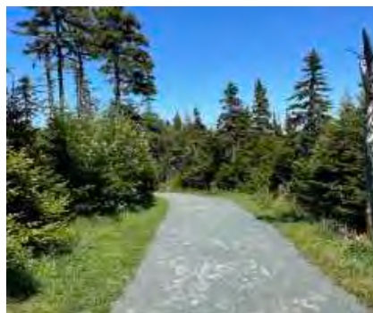
Level, well-graded granular trails can meet accessibility guidelines, trails do not necessarily have to be paved
