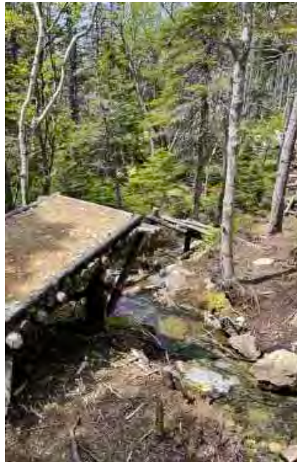
Mountain biking infrastructure at Skinners Road
