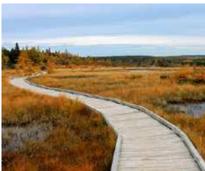
Boardwalk with side barriers to improve accessibility (Parks Canada)
