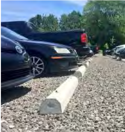
Precast concrete curbs used to delineate parking spaces in a granular parking area (Pinterest)
