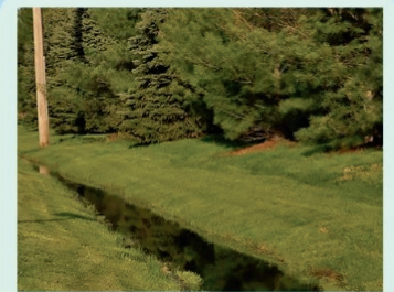
Image 1.2 demonstrates a well managed and maintained roadside ditch. Clean flowing water and healthy riparian vegetation shows that this is a well functioning waterway.
