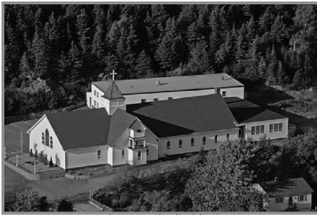
St. Lawrence Anglican Church Complex Portugal Cove, Newfoundland
